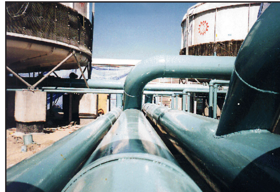
Cooling water pipes coated with ARC S2
